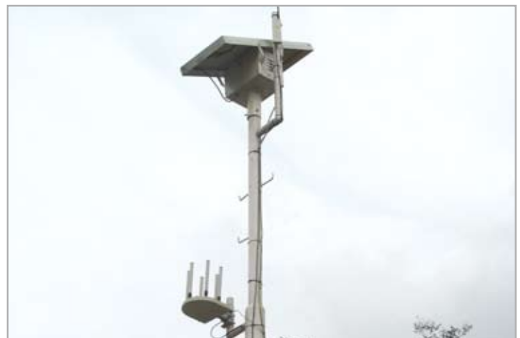
Solar-powered WBS-2400 base station
