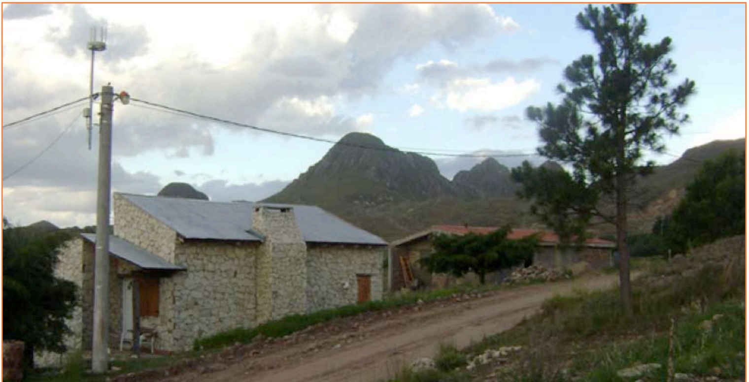
Typical village coverage in rural San Luis
